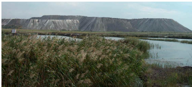
Fig. 1 Waste landfill in operation
